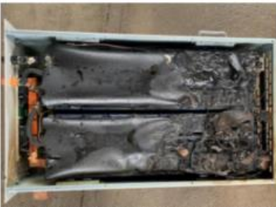
Figure 28e. Photo 04 of initiating module M20 after test.
